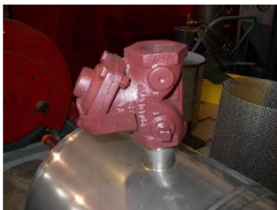
Figure 8: Flush valve
