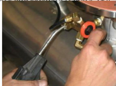
Figure 40: Blowing out air lines
