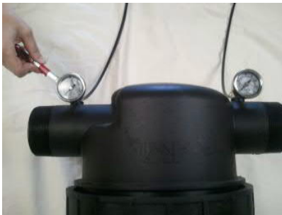
Figure 18: Removal of pressure gauge
