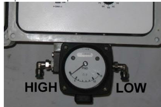
Figure 3: High & low-pressure ports on the DP switch/gauge
