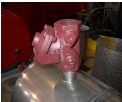
Figure 20: Flush valve
