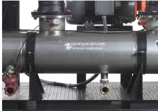
Figure 2: Saddle type filter support
