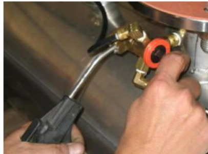
Figure 32: Blowing out air lines
