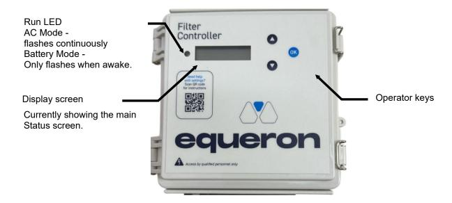
The controller has a list of menu items that allow adjustment of the filter back flushing. The menus are accessed by pressing the "UP" or "DOWN" keys.
